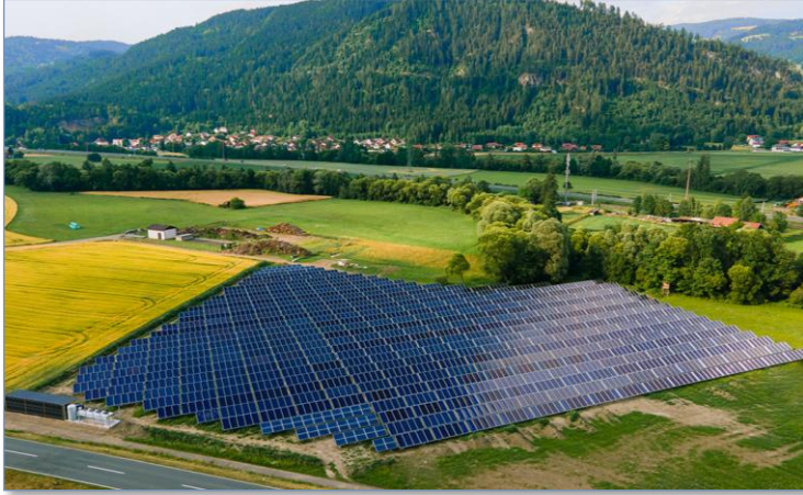
Friesach, Source: Solar Engineering Guggenberger
